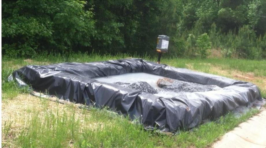
1. Concrete washout will be collected and retained so that this caustic material does not reach the soil surface and then migrate to surface waters or into the ground water. Any form of concrete washout collection is acceptable, as long as it is effective.
